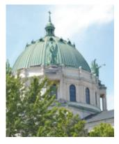
As you know, Buffalo's harsh climate has taken its toll on the Basilica's dome over the past 100 years and water infiltration has significantly damaged the plaster and interior paintings.
